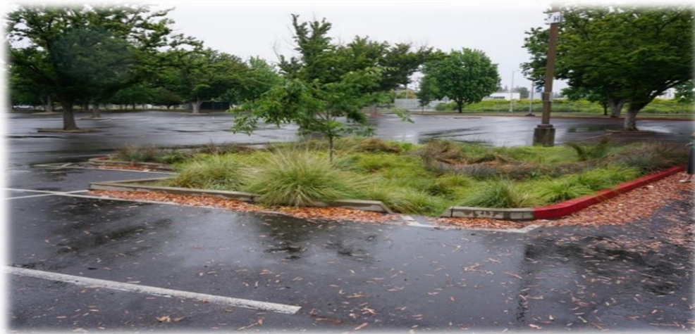
Figure A: Photograph of a Bioretention System at Sacramento State University
